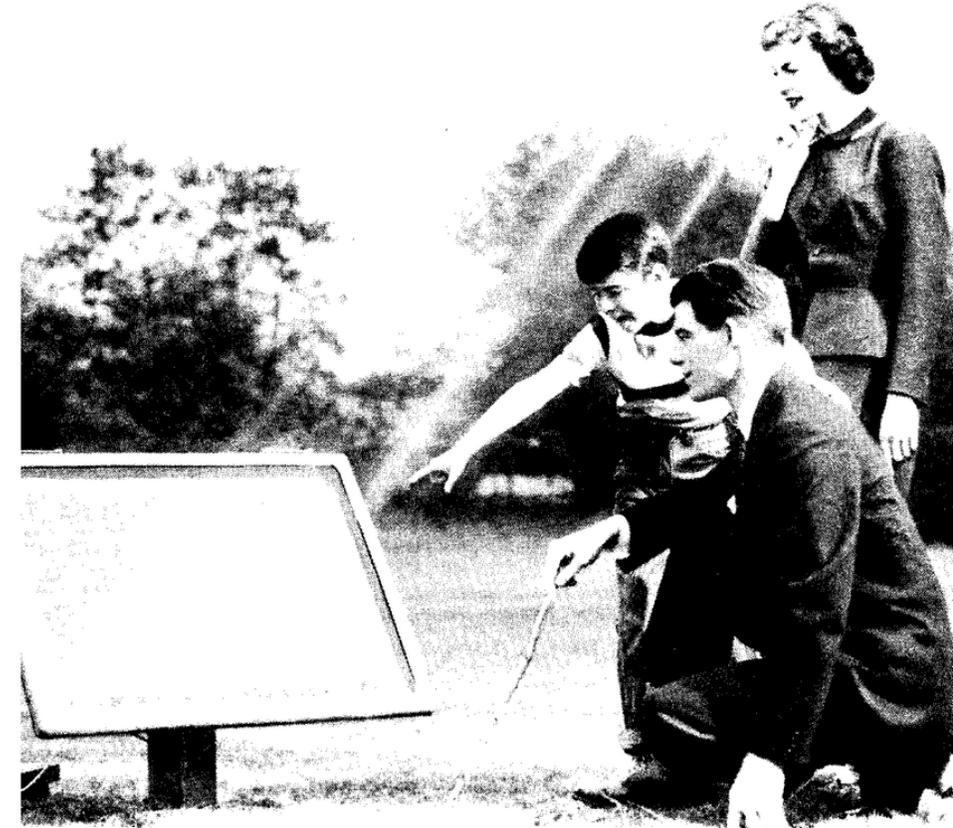
**Something New Under the Sun.** It's the Bell Solar Battery, made of thin discs of specially treated silicon, an ingredient of common sand. It converts the sun's rays directly into usable amounts of electricity. Simple and trouble-free. (The storage batteries beside the solar battery store up its electricity for night use.)
