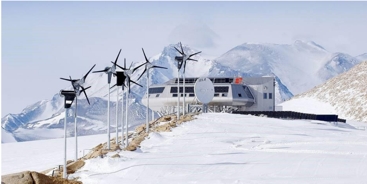
Fig.V.2. The Princess Elisabeth research station in Antarctica powered by a hybrid microgrid [44].
