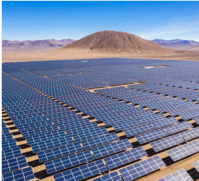
Fig.II.10. Photovoltaic field (solar farm).
